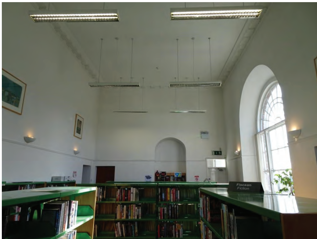
Plate 19 Room at first floor 2017
