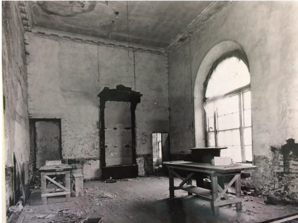
Plate 18 Room at first floor level in 1983
