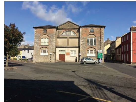
Rear southern elevation of building
