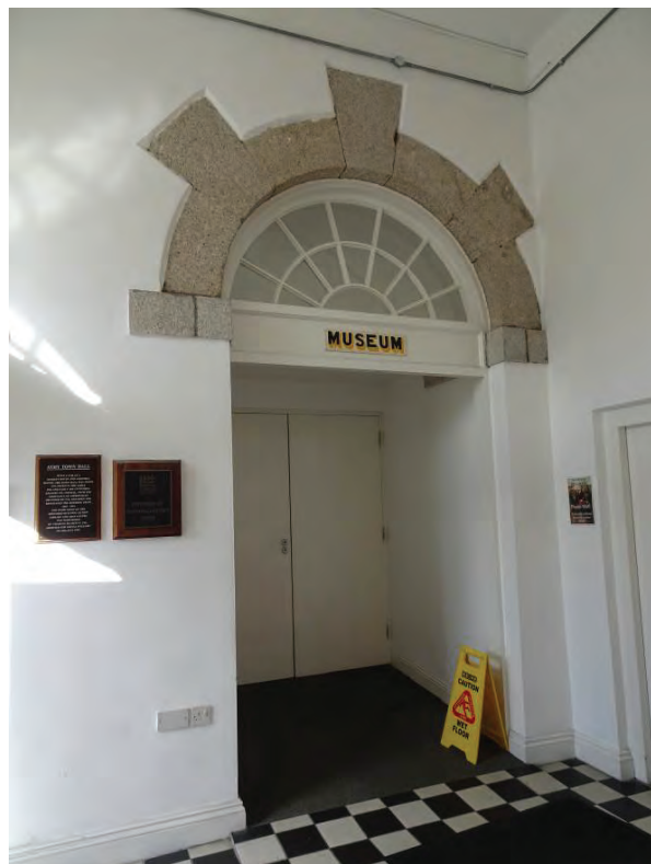
Plate 23 Original external door surround now incorporated into the interior of the building
