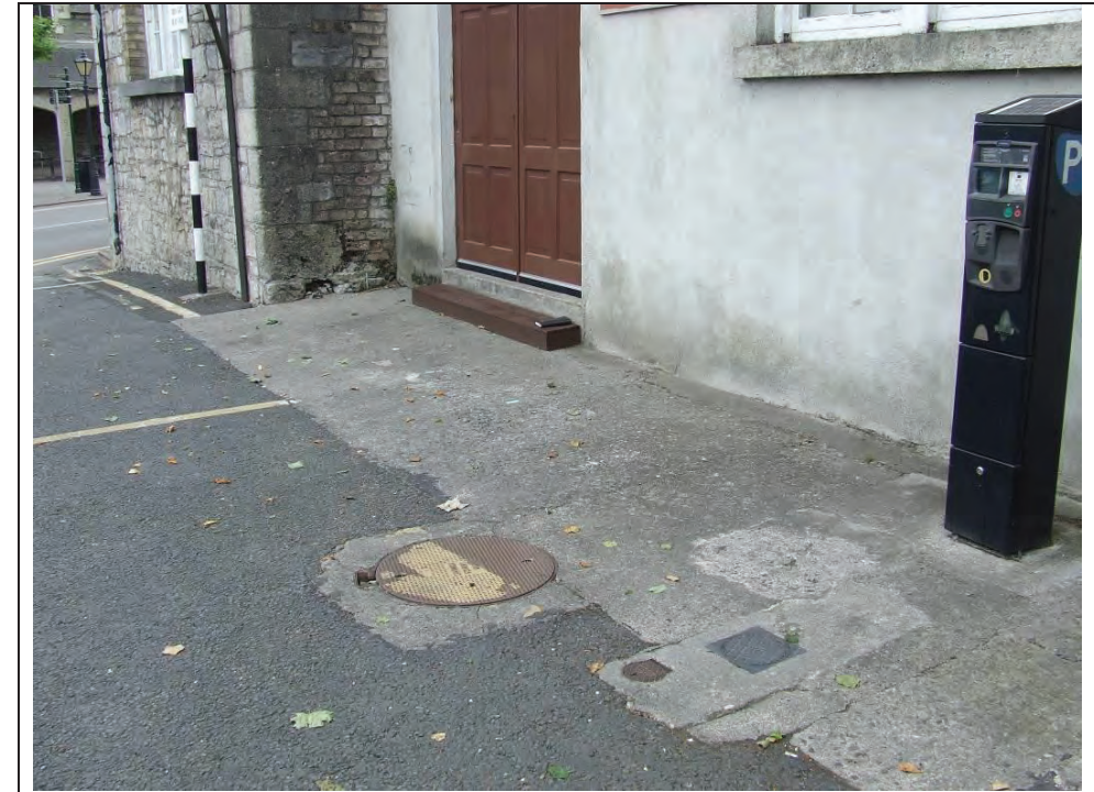
Plate 3 Showing existing services in proposed extension location, facing northwest.
