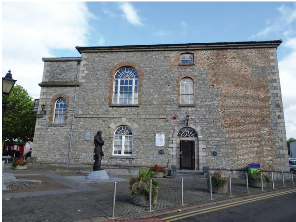
Plate 7 West elevation in 2017. Note the two chimneys and external render have been removed.
