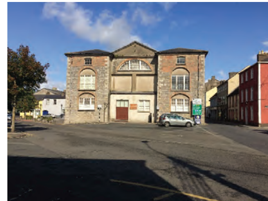
Rear southern elevation of building
