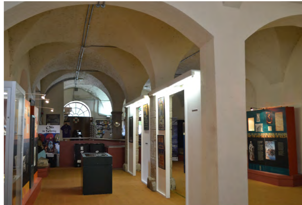
Image 18: Groin vaulted central space looking North
