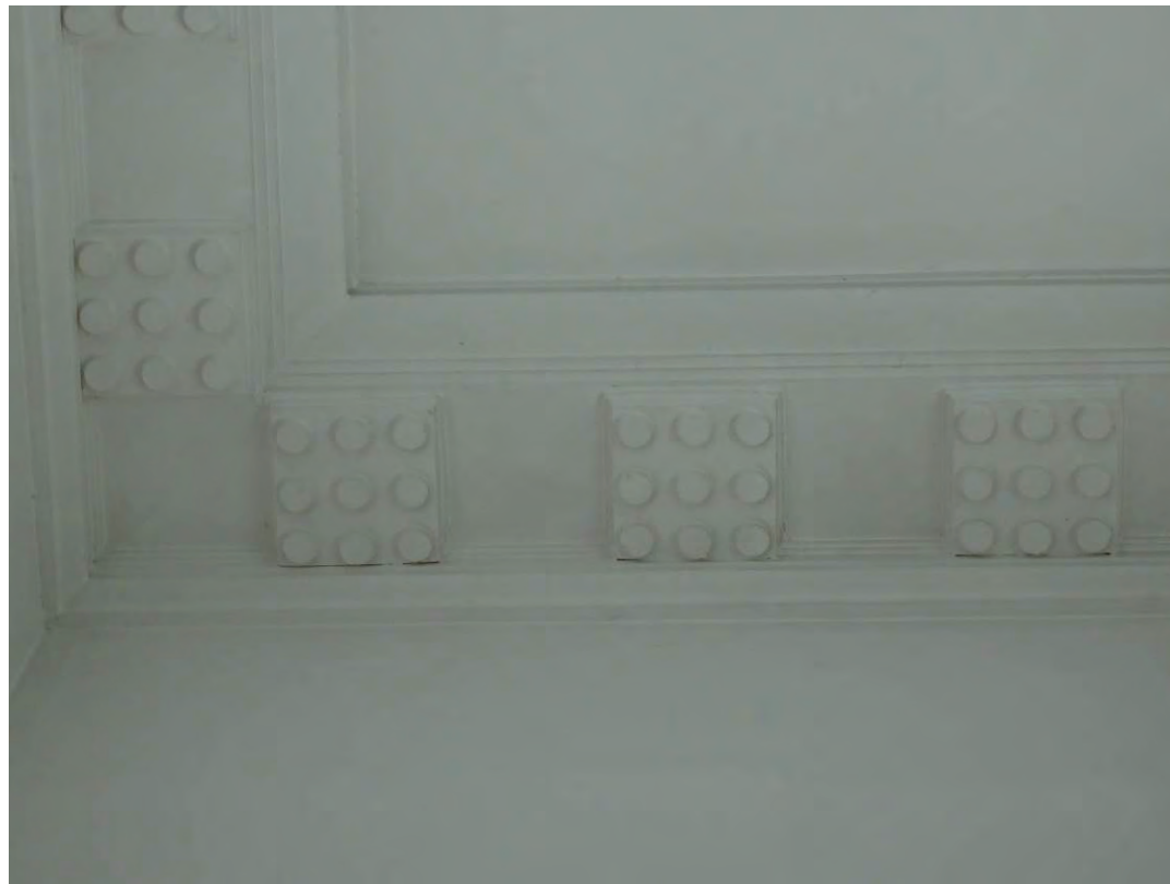
Plate 27 Doric cornice at first floor level is a recreation of the early 19 th Century cornice.
