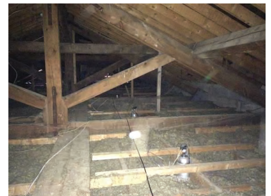
Accessible attic space with insulation visible
