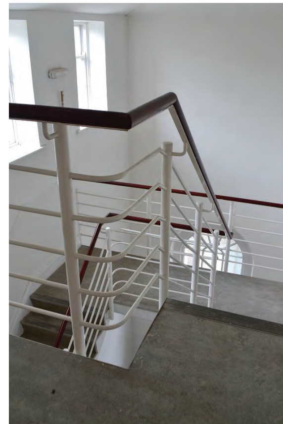
Plate 25 Staircase north-east side, dating to 1980s.
