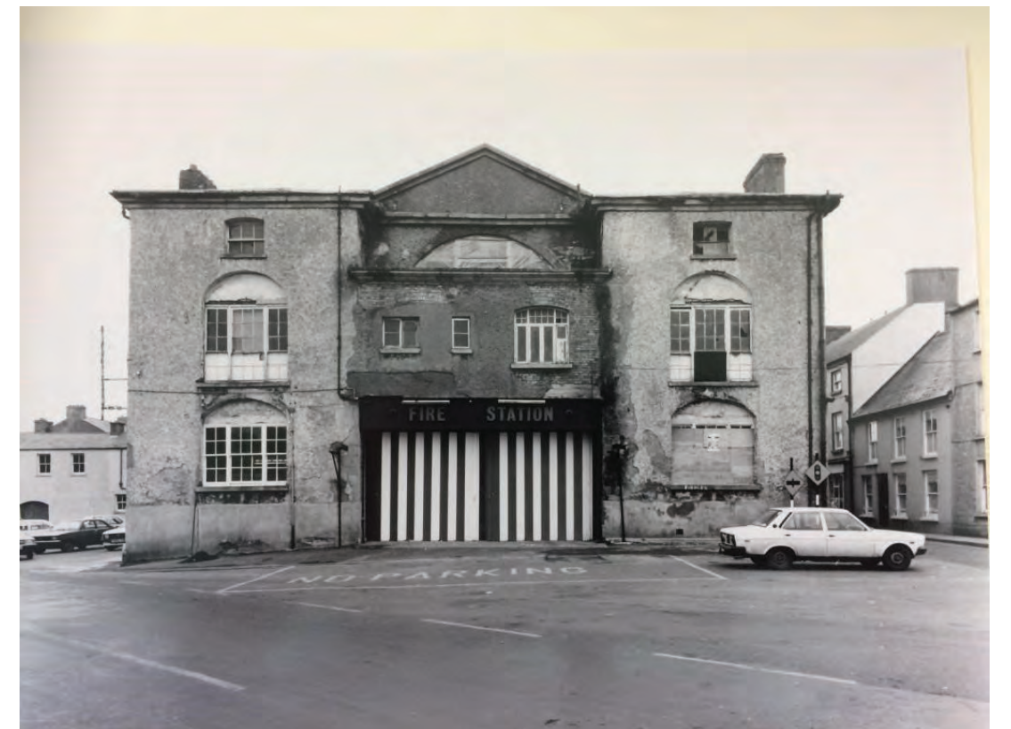
Plate 9 Rear (south) elevation in 1983 The rear elevation was removed at ground level to provide vehicular access for fire tenders.
