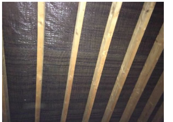
Accessible attic space showing beams and roof felt in good condition.
