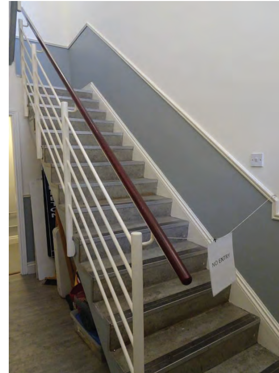
Plate 24 Staircase east side dating to 1980s.
