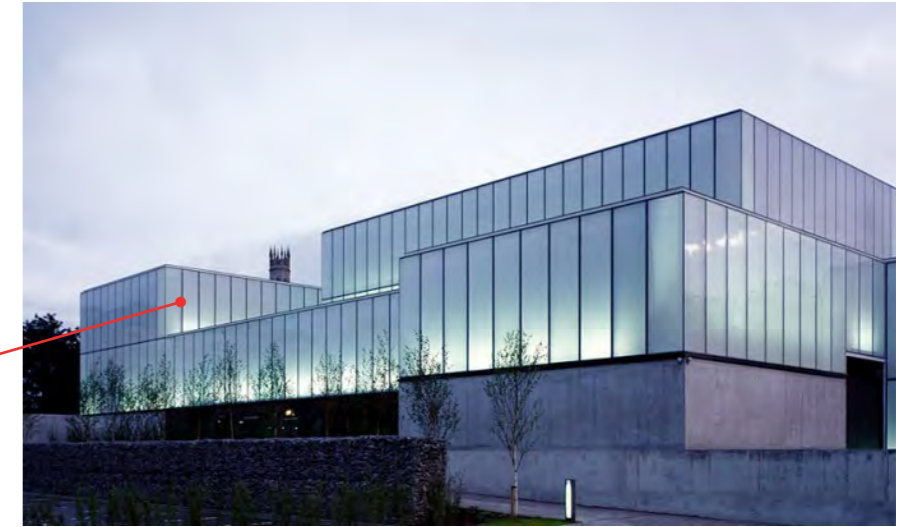
Image 61: Carlow Arts Centre, John Pawson: Translucent glazing
