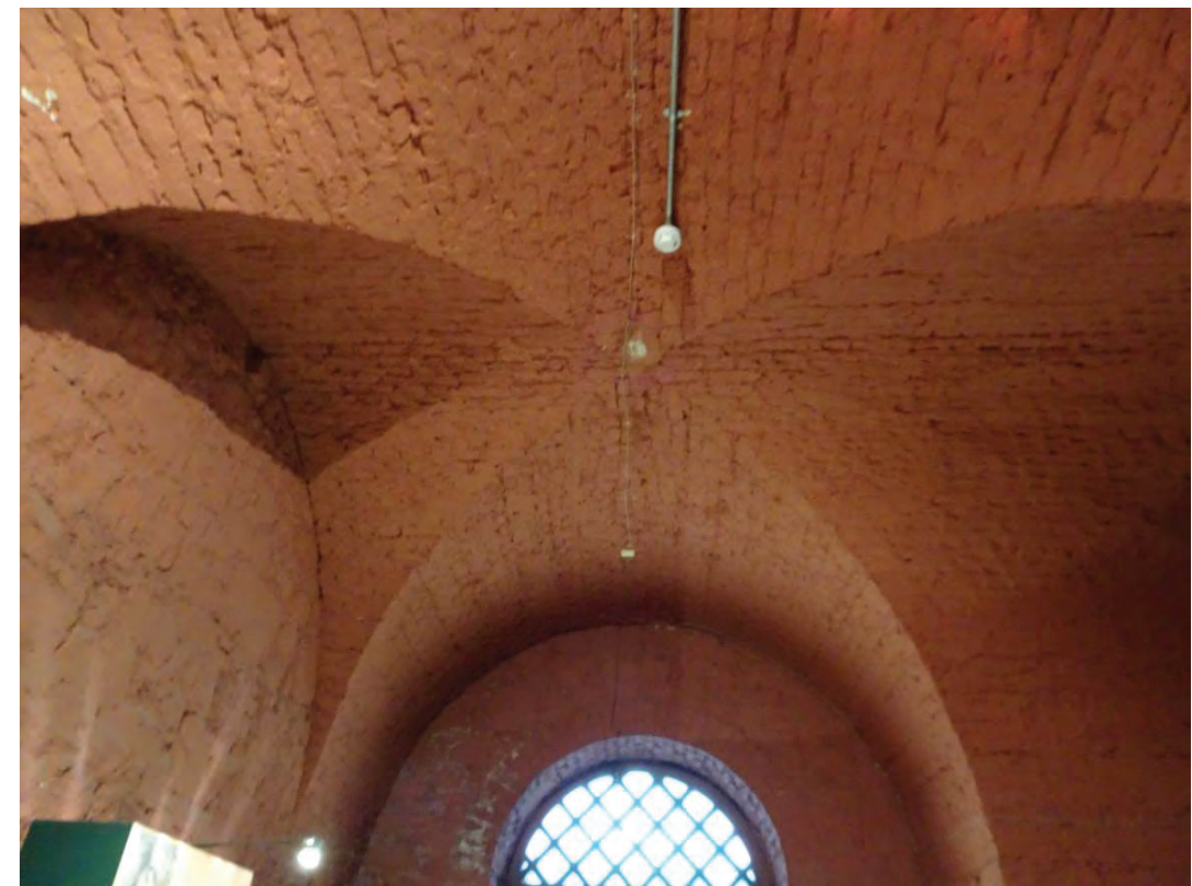
Plate 21 Original brick vaulting east side
