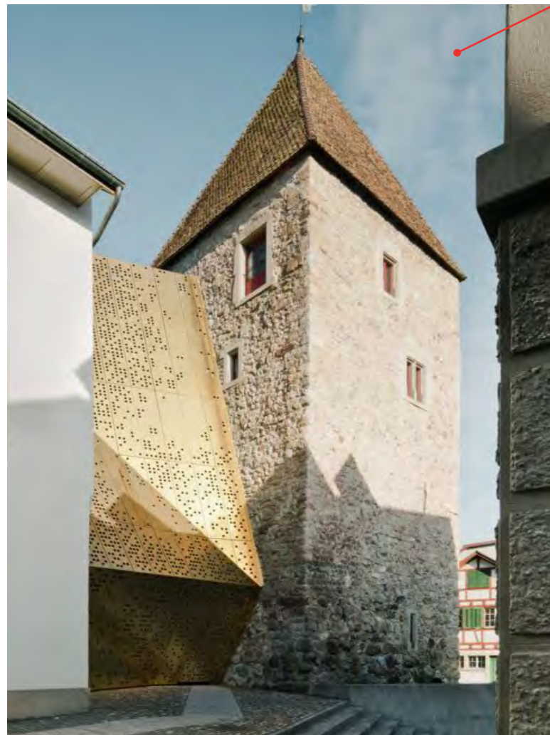
Image 58: Stadtmuseum Rapperswil, Switzerland: MLZD Architects Anodised steel cladding on a modern extension to a protected structure
