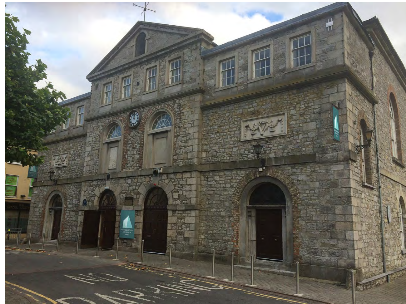
Image 65: Indicative signage on the North Facade
