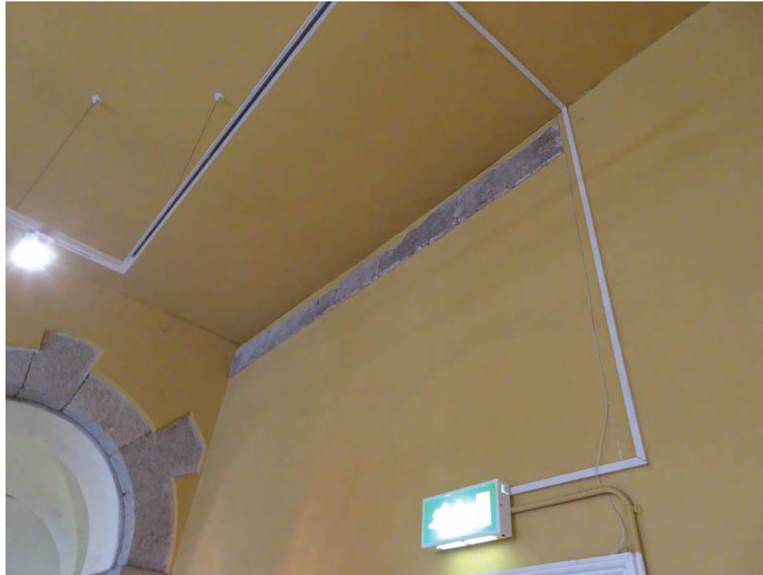
Plate 22 Original external door surround and string course now incorporated into the interior of the building
