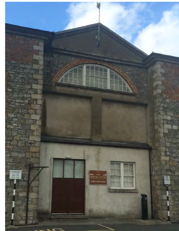
Image 15: Central bay of South facade.
