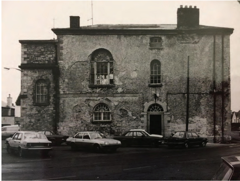
Plate 6 West elevation in 1983 before refurbishment work commenced.
