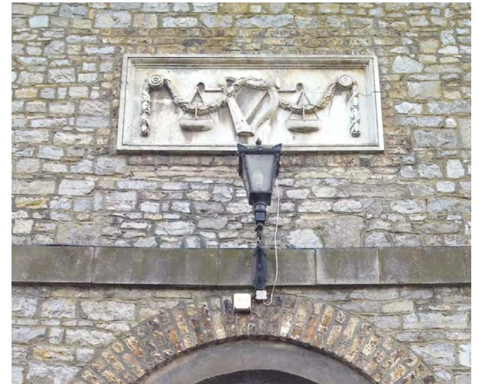
Image 16: Carved Frieze above Door on North Facade
