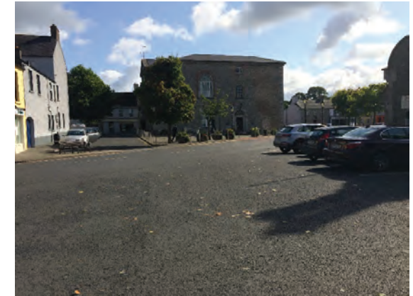
Western elevation of building
