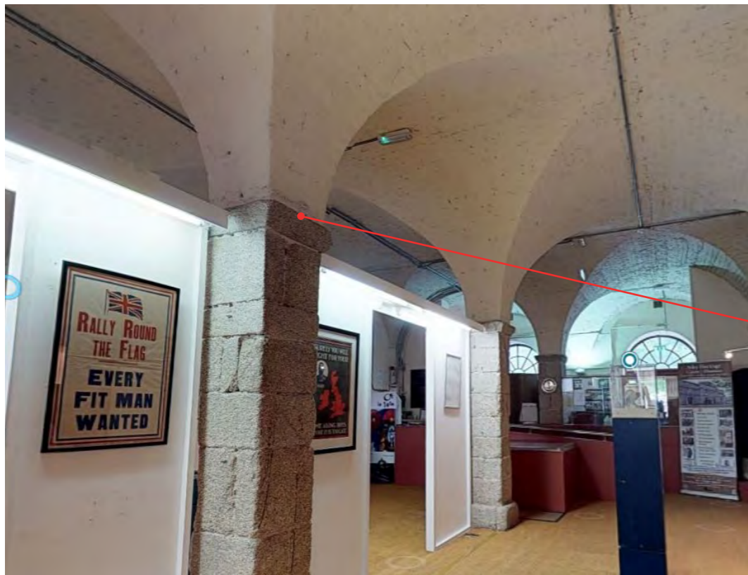
Image 69: Existing ground floor groin vaulted space
