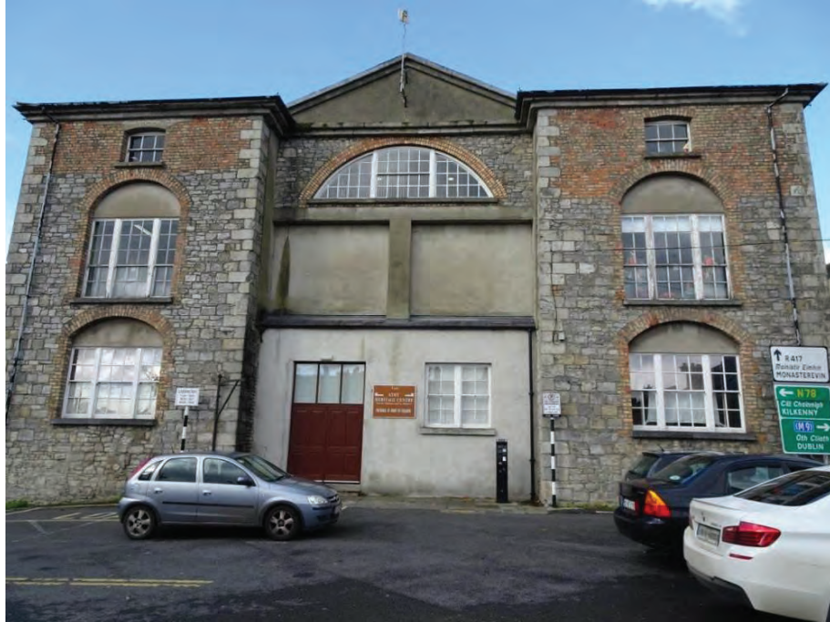
Plate 10 Rear (south) elevation in 2017. The overhanging section at first floor level was removed and the ground floor entrance was altered when the fire station was relocated.
