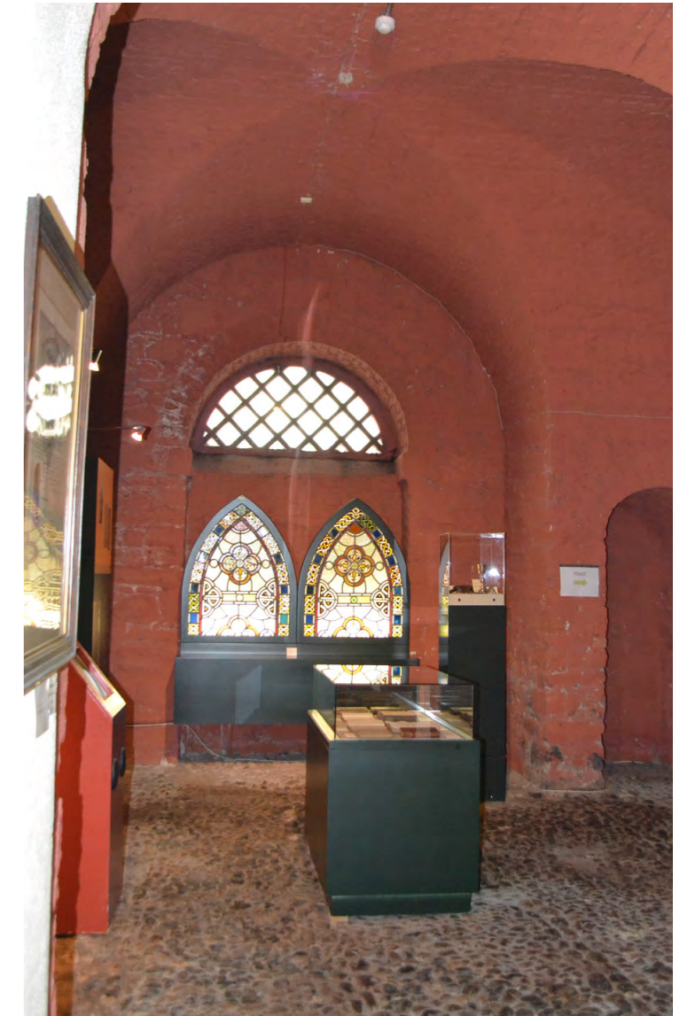
Image 22: Groin vaulted bay to East facade with cobblestone floor
