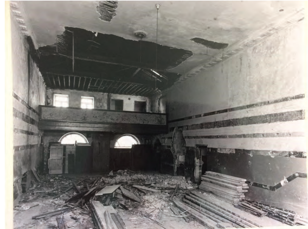
Plate 16 First floor space in 1983 looking north, before refurbishment works commenced. The balcony and four windows at second floor level were added in 1913.
